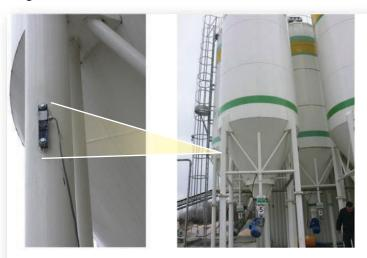
Installation of Silex sensors on round silo legs using weld tabs. Through-hole mount is used on H and L-section legs. Almost all leg types are suitable for Silex sensor installation.
